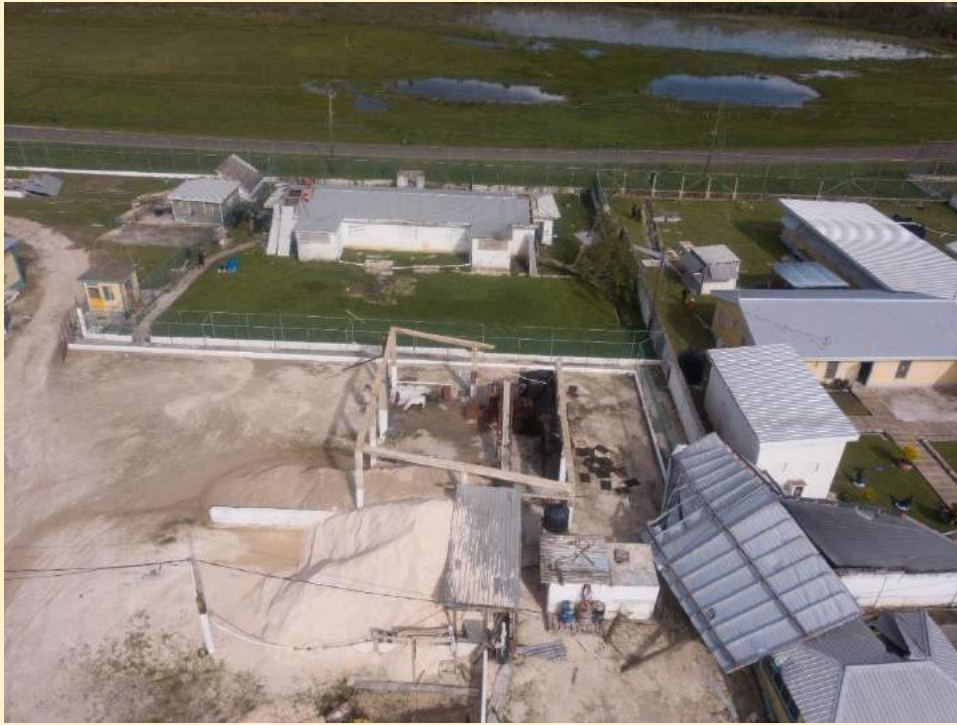
Block Factory demolished by Hurricane Lisa
